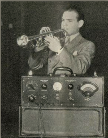
Charlie Teagarden (1913-1984) tests an early Silvertone trumpet using the Burgess "Acoustimeter", which was one of the first sound level meters invented. Subsequent advertisements for the Silvertone cited these tests as proof of the superior sound projection of its sterling silver bell.
