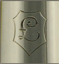
The bell of the Silvertone model is stamped with the English pound sterling symbol to indicate that it is made of sterling silver. Sterling silver is an alloy most often made of 92.5% silver and 7.5% copper. The copper is needed to strengthen its durability, and in this instance its acoustical advantage compared to brass.
